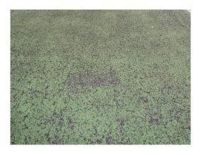
The existing court surfaces indicates no signs of sub-base cracking, heave or displacement.
