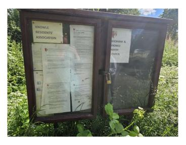
The current noticeboard has display of 92cm x 120cm and can fit a maximum 6 sheets A4 each side at a push. It is difficult to push pins into, has water ingress and insects living inside. The verge around it is also not being maintained.
